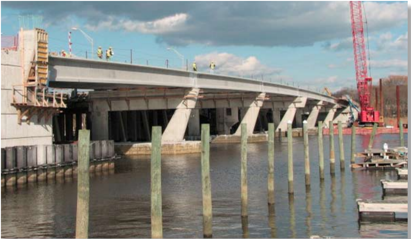
The Stage 1 eastbound structure under construction.
