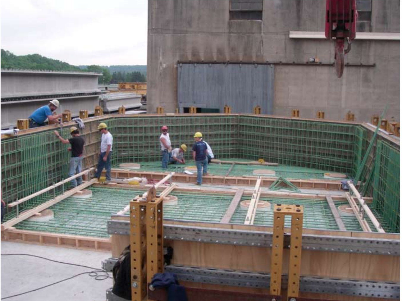
Placing reinforcement and setting forms for a precast concrete cofferdam.
