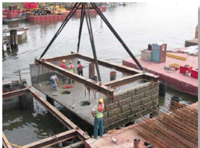
Precast cofferdam section being lowered into place.
